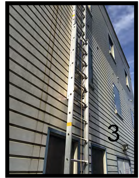
Ladder should be fly section in against the building next to desired location
