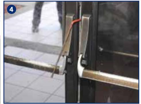
(2) A hook fashioned from ridged wire opens double doors. (3-4) A paint roller inserted between double doors actuates panic hardware.
