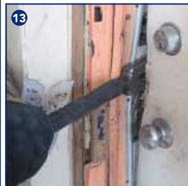
(11-13) The fork, with the bevel away from the door, is driven between the tight-fitting steel inward-swinging door and the jamb. Note that the deadbolt is beginning to fail.
