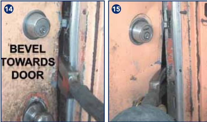
(14-15) After crushing the door and jamb, the fork is rotated so that the bevel is toward the door. The deadbolt fails when the shaft is pushed toward the door.
