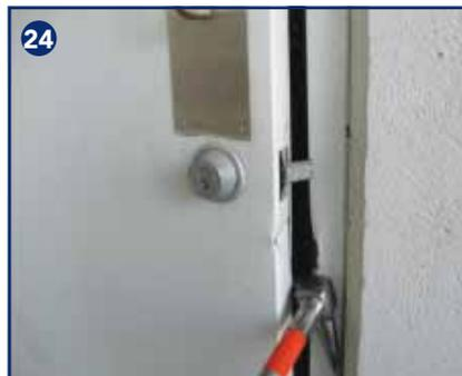
My confidence changed to embarrassment when we failed after repeated attempts. We later found that this door had large masonry nails driven into the edge on the hinged side. When closed, these nails fit into holes drilled into the doorjamb. I was naive to think that a businessman would spend a lot of money on a heavy door and several locks but leave the hinges vulnerable.
