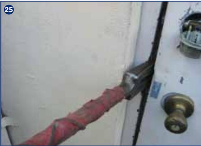
(25) The prying action of the fork is restricted in this outward-swinging door recessed in a concrete block wall.
