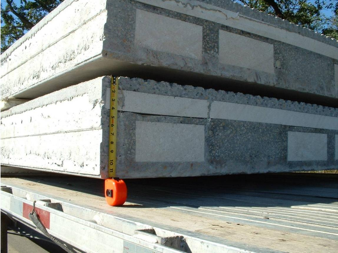
Wall panels used in the interior of a building are usually not insulated and may be manufactured with round or oval empty cores similar to those used in prestressed concrete floor plank.
