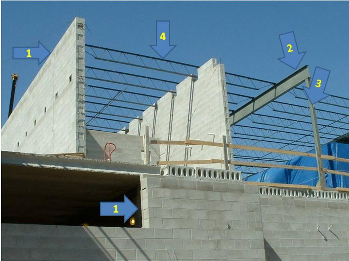
Photo 1 shows part of a school building under construction. The failure of primary structural members or of the connections between them can cause the collapse of the building or a part of it. Primary structural members are those without which the structure will not stand. They include load-bearing walls (photo 1 numbers 1, 1), columns (photo 1 number 3), and girders (photo 1 number 2, including ridge-boards and the trimmer/header assemblies that support stairways).
